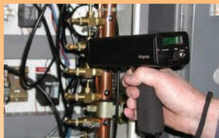
Detect air leaks
