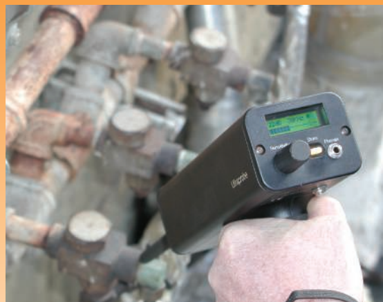
Inspect steam traps
